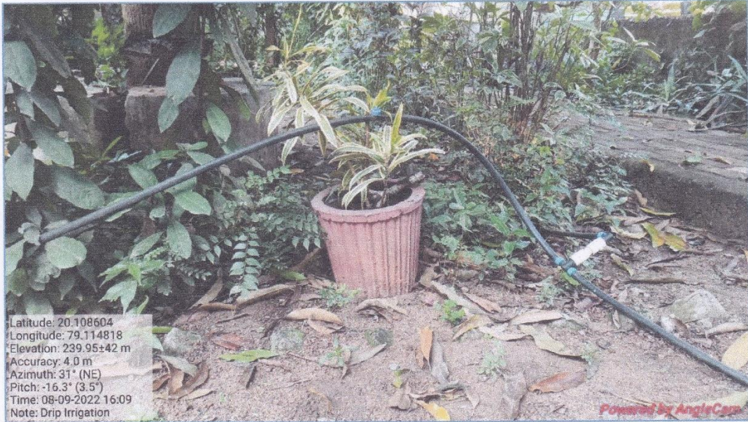
Drip Irrigation System in Botanical Garden
